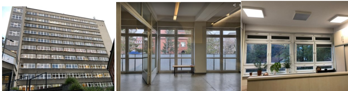
Figure 23: The office building-case study for the students at the summer school. A. Northern Façade with a connector to Main Building. b. View from the building 2 nd floor with western exposition c. View from the office on the 1st floor toward the northern side and greenery.
