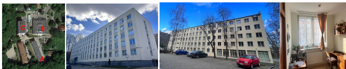
Figure 22: The dormitory building (A)- case study for the students at the summer school.
